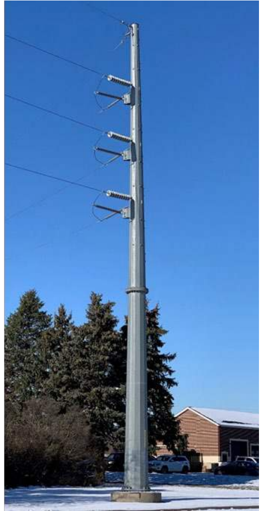
Figure 8 Photos of 115-kV Transmission Structures
