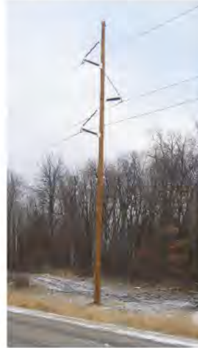
Typical 115-kV braced-post structures.
