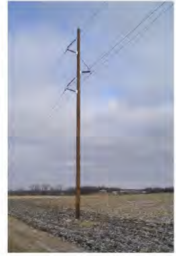
Typical 115-kV braced-post structures.
