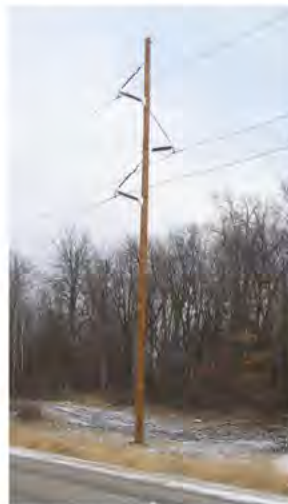
Typical 115-kV braced-post structures.
