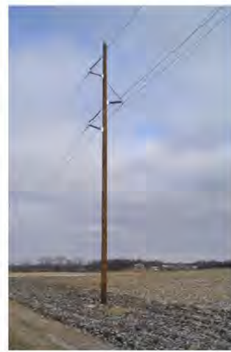
Typical 115-kV braced-post structures.
