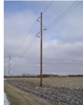
Typical 115 kV single circuit H-braced post structure
