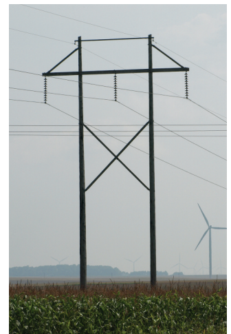
230-kV/345-kV H-frame transmission structure
