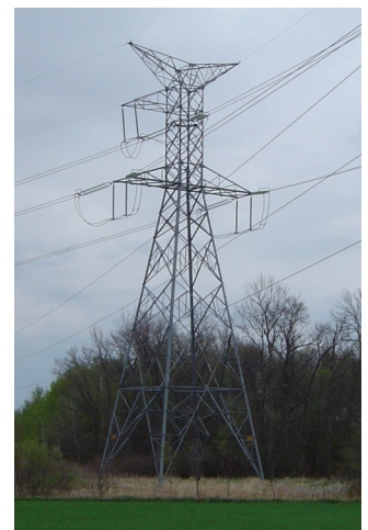
230-kV/345-kV lattice transmission structure
