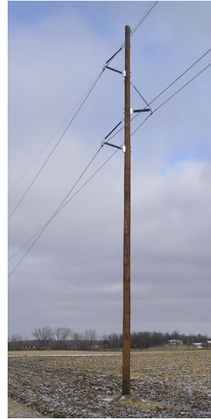
Typical 115-kV structures
