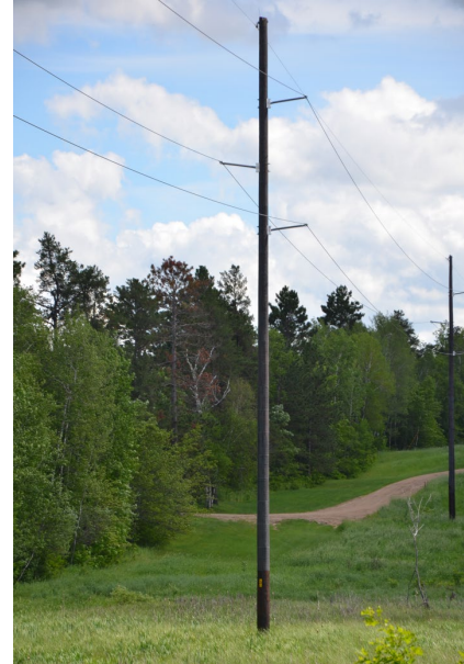
Typical 115-kV circuit
