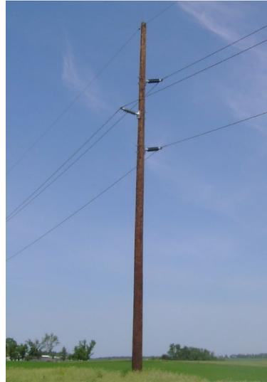
Typical 69-kV single circuit
