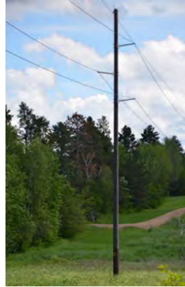
Typical 115-kV wood single circuit structure with and without distribution under build.
