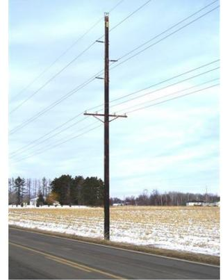
*Typical 69-kV wood double circuit structure with distribution underbuild*
