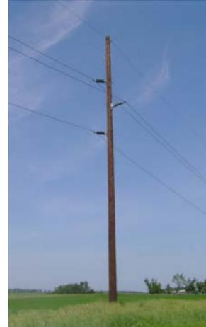
*Typical 69 kV wood single circuit structure*
