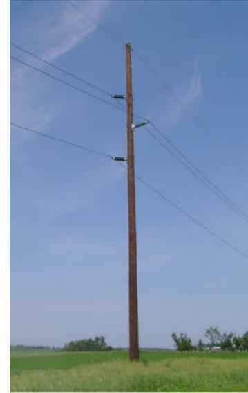
*Typical 69-kV single circuit structure*
