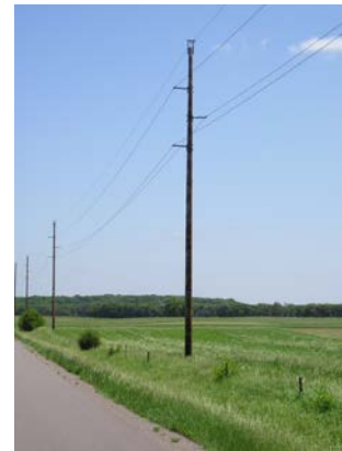
Typical 115 kV wood single circuit structure
