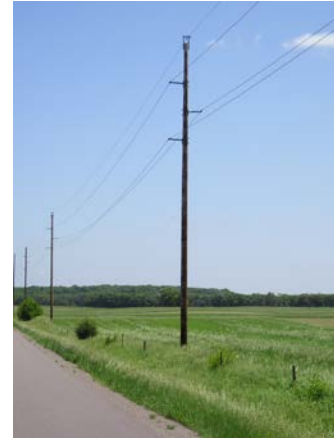
Typical 69-kV Circuit
