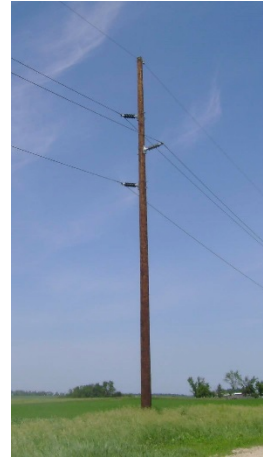
Typical 34.5-kV wood single-circuit structure
