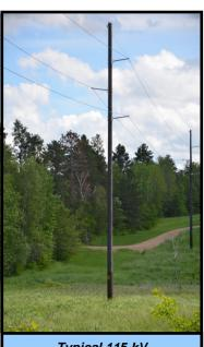
Typical 115 kV Transmission Structure
