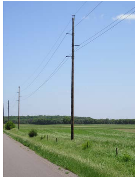
Typical 69-kV Circuit
