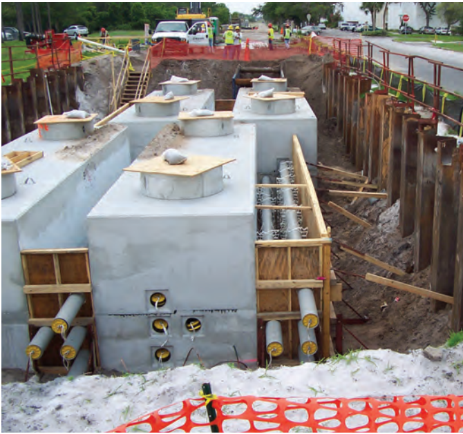
Splice boxes and manholes must be installed every 1,500 to 2,000 feet to allow for regular inspection and maintenance.
