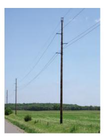
Transmission lines, such as those Great River Energy builds, deliver large or "bulk" amounts of electricity. Pictured is a common structure for 69-kV and 115-kV transmission lines. energized – even without actually touching the power line – an arc of electricity can form in the air connecting the two and cause very serious burns. Arcs heat the air around them to up to four times the surface temperature of the sun. Serious burns are not uncommon even 10 feet from an electric arc.
