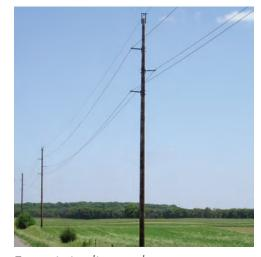
Transmission lines and structures are usually smaller than landowners expect at first. The large lattice towers that come to mind are rarely used any longer. Pictured above is a common structure for 69-kV and 115-kV transmission lines.
