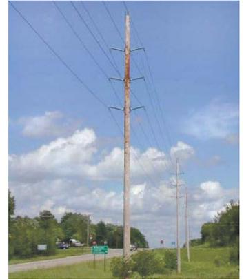
*Typical 115-kV wood double circuit structure without distribution underbuild*
