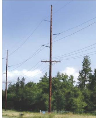
*Typical 115-kV wood single circuit structure with distribution underbuild*
