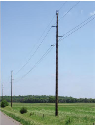
*Transmission lines, such as those Great River Energy builds, deliver large or “bulk” amounts of electricity. Pictured is a common structure for 69-kV and 115-kV transmission lines.*
