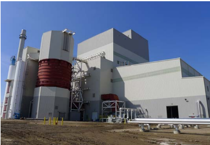
Spiritwood Station uses Best Available Control Technologies to control emissions.
