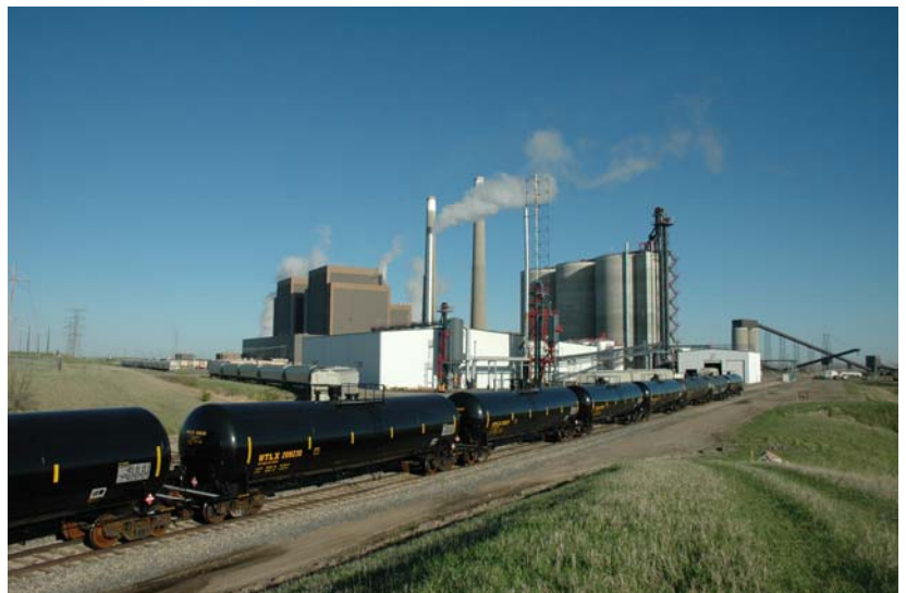
Blue Flint Ethanol with Coal Creek Station in the background.
